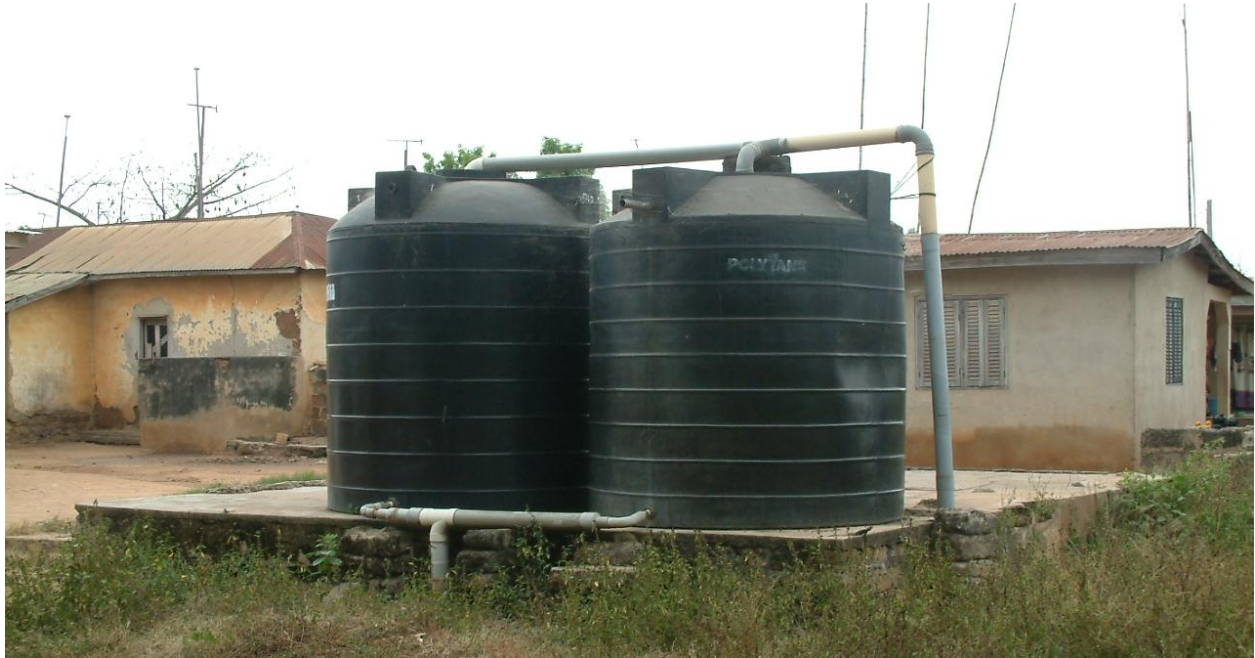
Figure E3: Current two 2,000 gal storage tanks in village, note the size of existing concrete support structure is made to support additional tanks.
