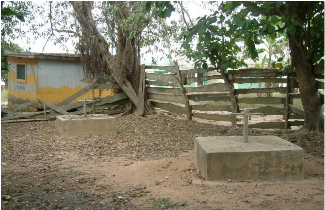
Figure E4: Current water distribution site in village. Currently not in use because of nonexistent pump.
