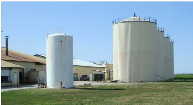
Fair Oaks Dairy farm digester in Indiana, USA
