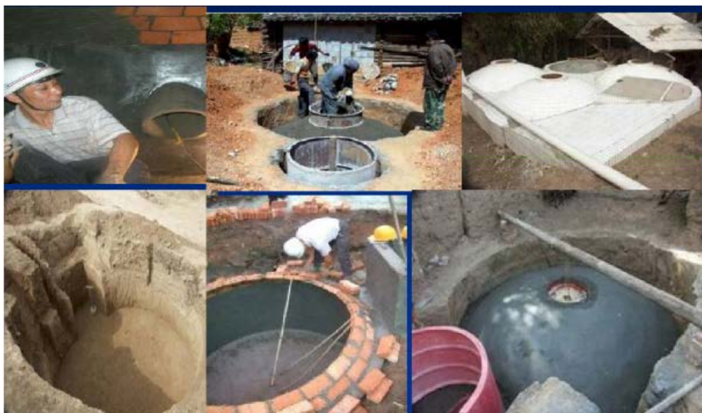
Biogas digester in construction
