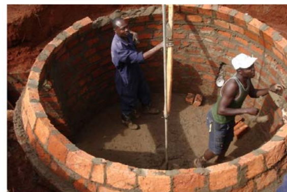
Fixed-dome digester under construction in Kenya
