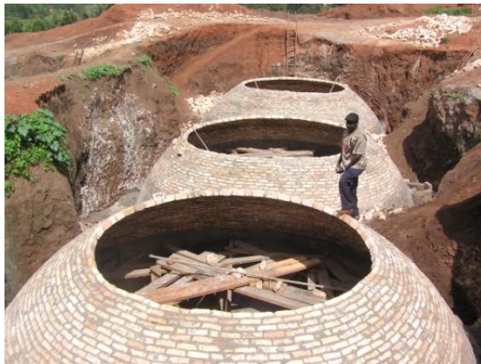
Biogas plant under construction Kitarama prison, Rwanda.
