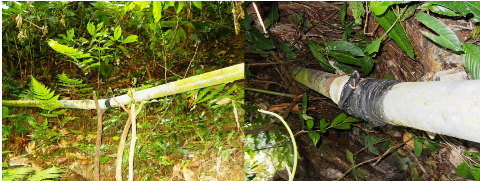
Picture: Current condition of conduit
