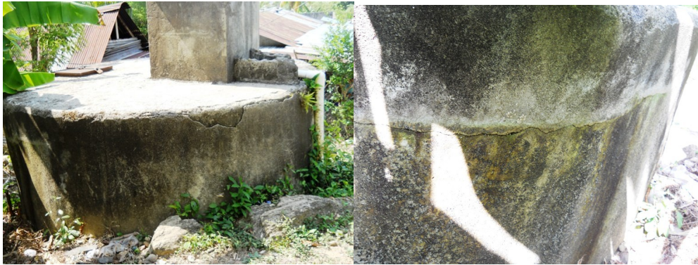
Picture: Current state of tank
